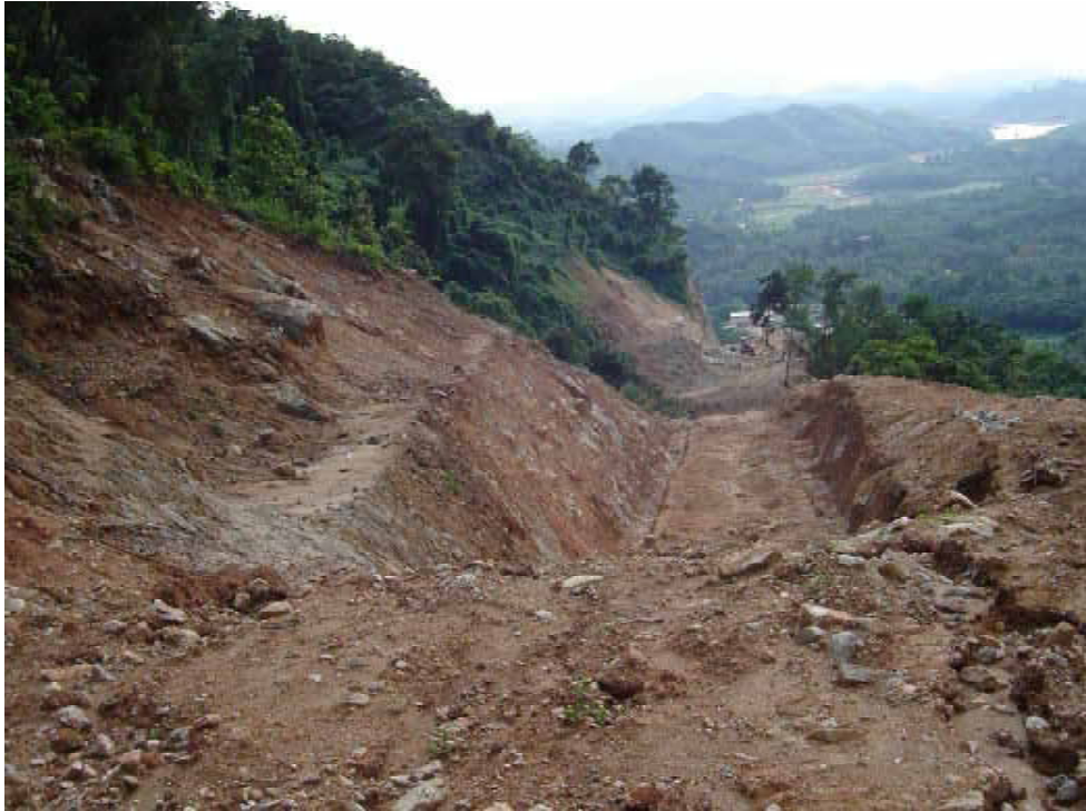
Picture 1 Excavations for Penstock track on a slide zone.
